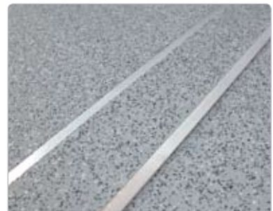
Typical example: AVR5020 repairing safety flooring.
