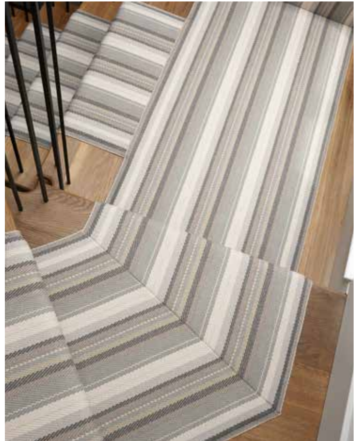
Isis Reed mitred on a long winding step and overlaid on landing
