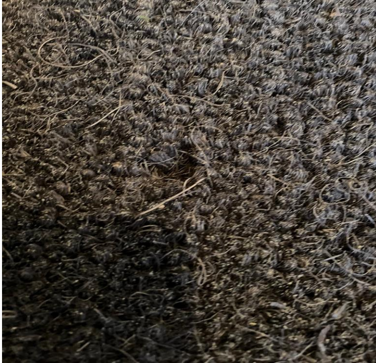
Tufting issue in coir matting – requires replacement
