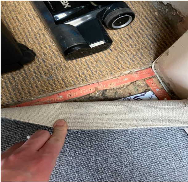
Carpet at top cupboard landing to be trimmed back and installed into gripper rods neatly
