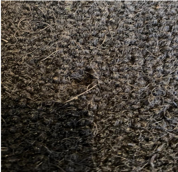
Tufting issue in coir matting – requires replacement
