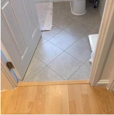
Landing To Tiles Bathroom
