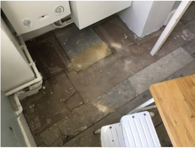
Kitchen Concrete Patch
