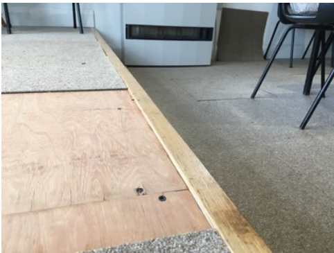
Raised Platform Area
