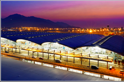
Hong Kong International Airport
