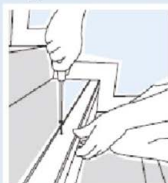
Unfilled stair nosing channel fixed to step.
