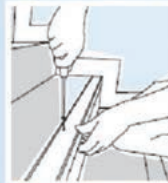
Unfilled stair nosing channel fixed to step.
