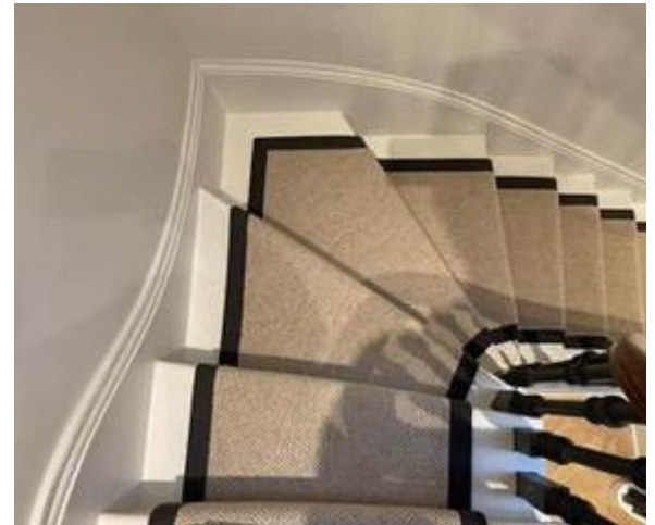
Fixed Perimeter: the runner has a fixed perimeter from the edge, which means the width of the carpet varies around corners and bends. The marked B is the width of the perimeter between the runner and the edge.
