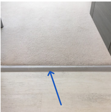
Bed 2 To Hall Remove ex Ali ramp & fit a Chrome S/Nap or a Chrome Zig Zag whichever fits best
