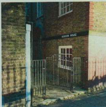
Entrance To Block
