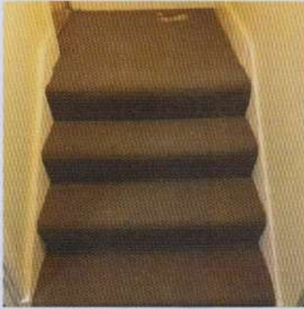
Replace Just These Areas on Common Stairs
